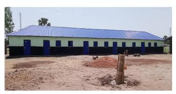
This structure is impressive. It is a total rebuild and built to a much higher standard. The doors and windows are all in place with strong locks on the doors and shutters for the windows. The internal walls are rendered and await painting. The builders are in the process of levelling the floor which will then be covered by a layer of mud bricks and surfaced with a cement screed. Finally the external rendering
